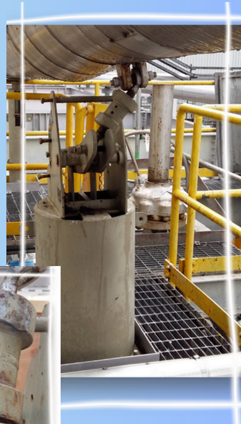
Damaged pipe supports
