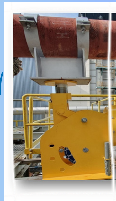
New pipe supports replaced
